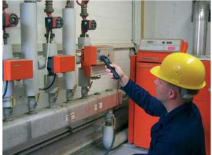
*Checking the temperature of heating circles*
